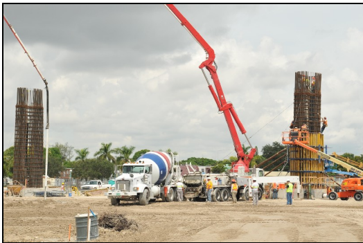
a) Super Columns Erected
