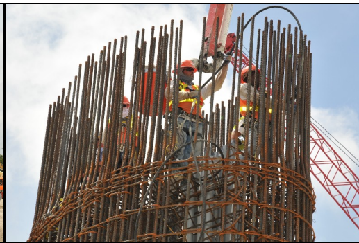
b) Workers Pouring Concrete
